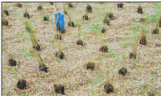
Newly planted Phragmites in gravel reedbed prior to increasing water level
